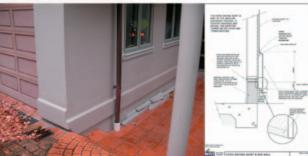
Concrete nibs are often installed in conjunction with Drying Skirts to address difficult clearance problems and minor timber stud damage.
