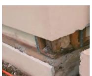
The existing cladding is cut away before installation, allowing timber inspection and replacement in the key locations around the perimeter of the building.
